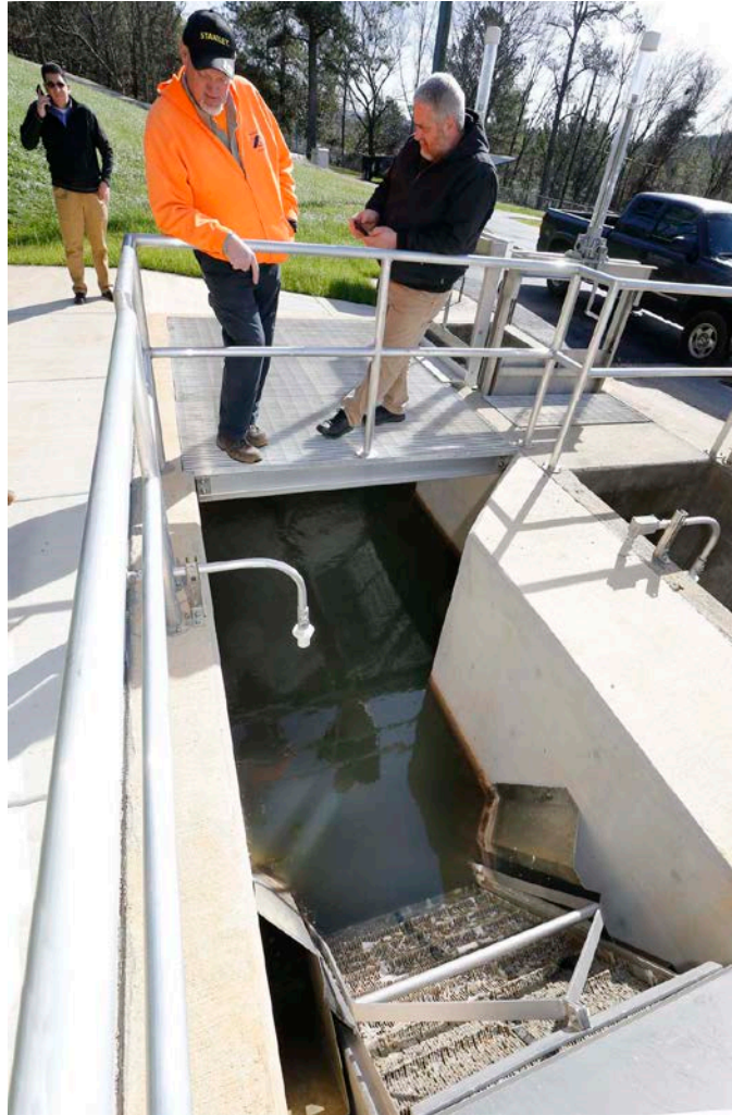
Anniston Water Works Manager, Ed Turner, Plant Maintenance Supervisor Steve Junior and Environmental Supervisor, David Henson look at debris trapped at the McClellan Waste Water Treatment Plant during a tour of the Anniston Water Works lift stations and treatment plant. Photo by Stephen Gross / The Anniston Star
