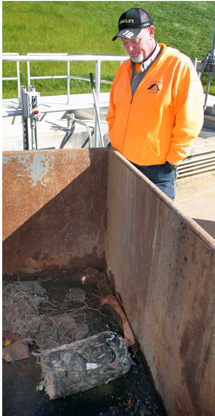
Anniston Water Works Plant Maintenance Supervisor Steve Junior looks at debris in a dumpster ready for removal at the McClellan Waste Water Treatment Plant during a tour of the Anniston Water Works lift stations and treatment plant. Photo by Stephen Gross / The Anniston Star
