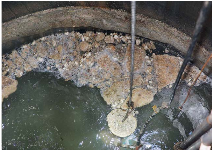
Grease and trash float to the surface in a holding tank at the Meadow Park lift station during a tour of the Anniston Water Works lift stations and treatment plant. Photo by Stephen Gross / The Anniston Star
