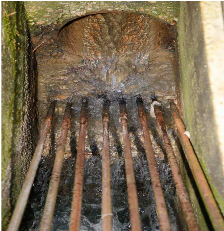
Water flows into the McClellan lift station during a tour of the Anniston Water Works lift stations and treatment plant. Photo by Stephen Gross / The Anniston Star
