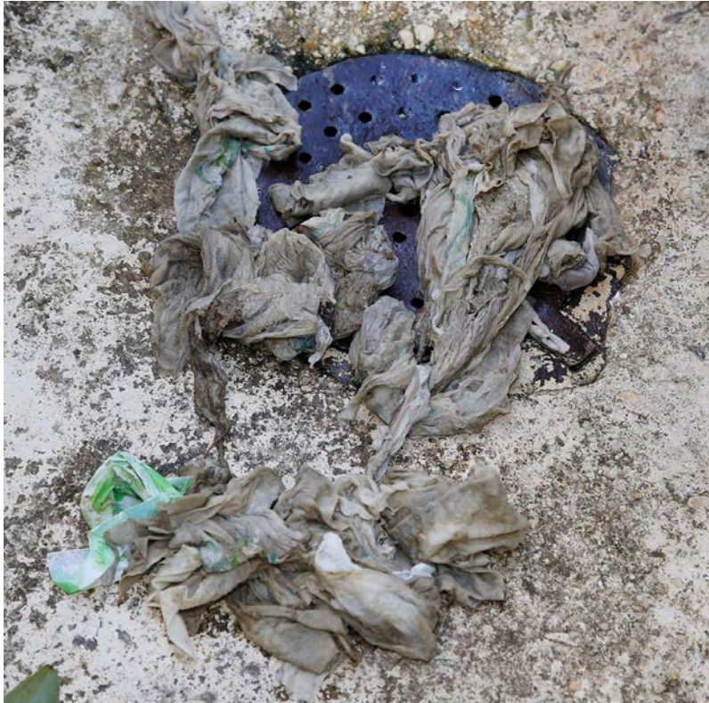
Flushable wipes that clog up the McClellan lift station system are in abundance during a tour of the Anniston Water Works lift stations and treatment plant. Photo by Stephen Gross / The Anniston Star
