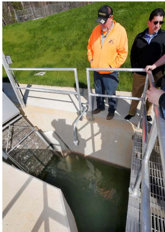
Anniston Water Works Plant Maintenance Supervisor Steve Junior looks at debris trapped at the McClellan Waste Water Treatment Plant during a tour of the Anniston Water Works lift stations and treatment plant. Photo by Stephen Gross / The Anniston Star
