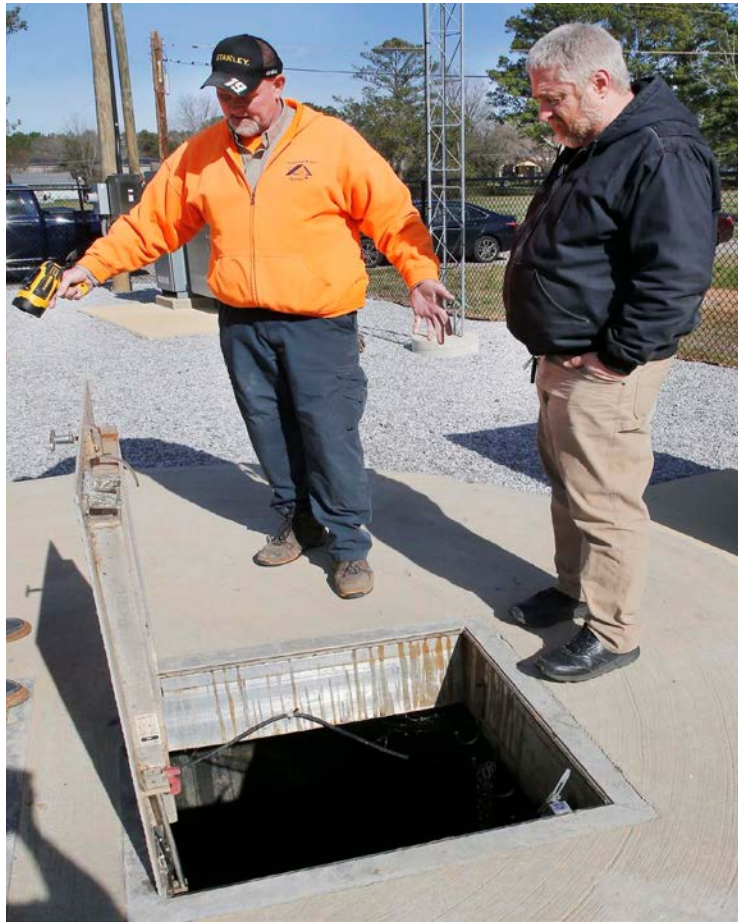
Anniston Water Works Plant Maintenance Supervisor Steve Junior and Environmental Supervisor, David Henson look at grease in the tank at the Meadow Park lift station during a tour of the Anniston Water Works lift stations and treatment plant. Photo by Stephen Gross / The Anniston Star
