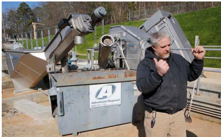
Anniston water Works Environmental Supervisor, David Henson describes how debris and grease clog up the works at the McClellan Waste Water Treatment Plant during a tour of the Anniston Water Works lift stations and treatment plant. Photo by Stephen Gross / The Anniston Star
